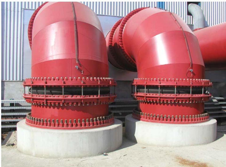
restraint compensator - design M DN 2600
